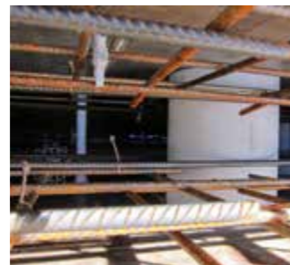
ZVR 200/300 in de bekisting vastgezet
